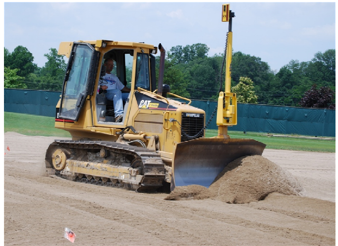
Spreading 85 / 10 / 5 Blend of Sand / AXIS / Soil
